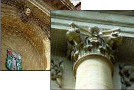
The Eastgate Portico in Gloucester has been sensitively covered with stone coloured netting, which blends well into the structure so that from a distance it is not noticeable. Although done to deter pigeons it gives a flavour of what can be achieved for gulls.
